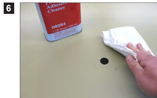
Using a quality adhesive removing solvent and a soft clean cloth to remove any of the remaining adhesive from the vehicle.
