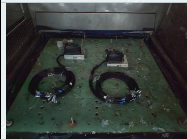
Fig.1-7 Sample installation (Transverse 1#,2#)
